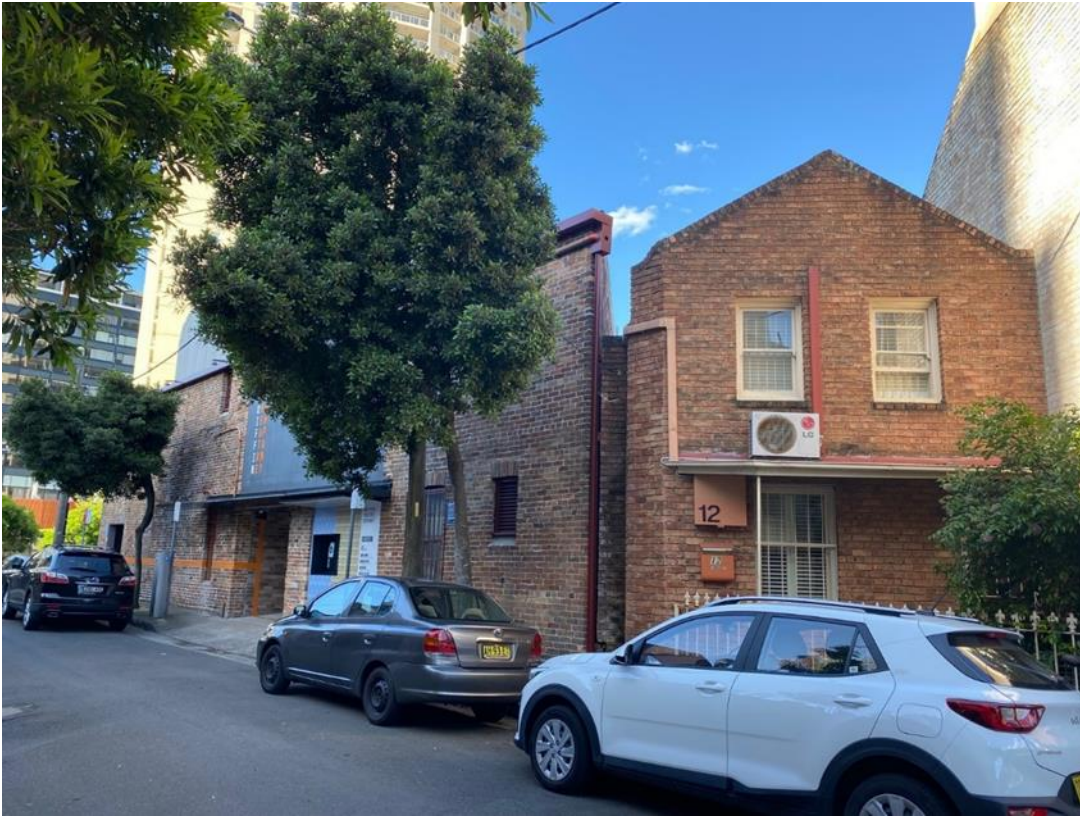
Figure 5: 10 and 12 Nimrod Street viewed from the south-west
